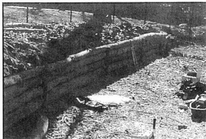
Retaining wall built from logs (by Roc Waters)
